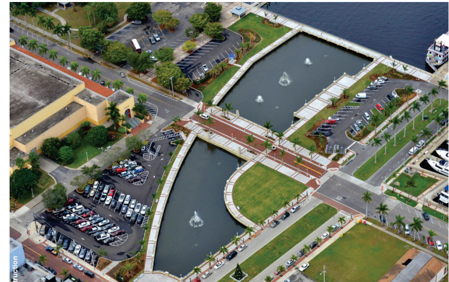
Downtown Detention Basin also improves Runoff Water Quality into Caloosahatchee River
