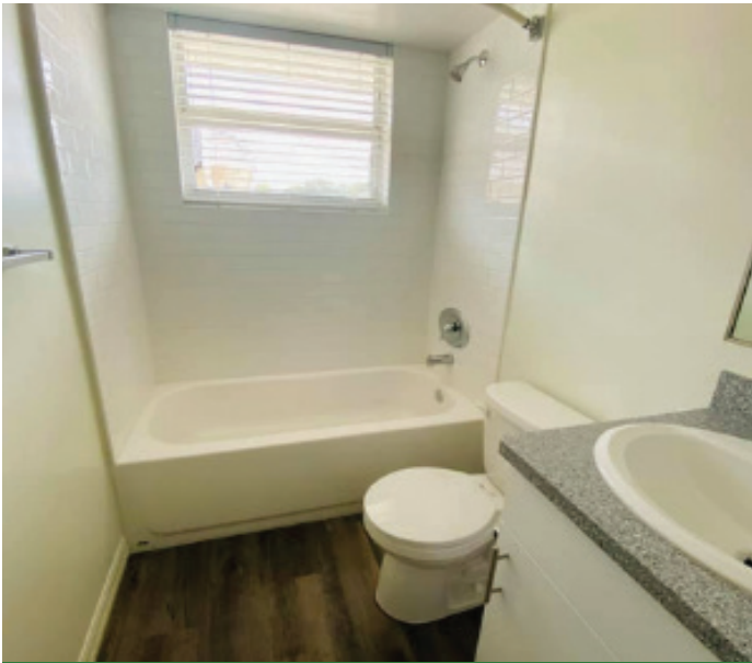
Bathroom Renovations Royal Palm Garden Apartments
