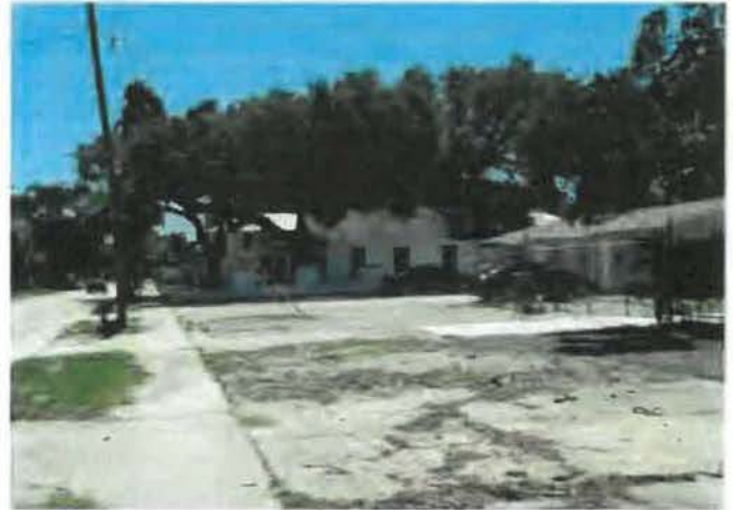
Deteriorating site conditions.
