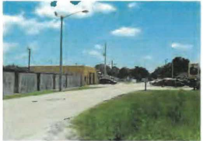
Lack of drainage and sidewalks, and deteriorating site conditions.
