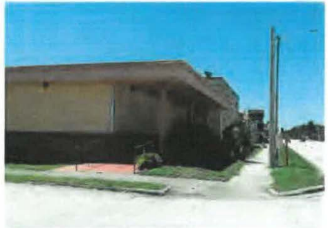
All windows and doors boarded.
