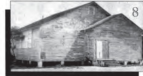
THE 1942 ADDITION TO THE WILLIAMS ACADEMY 1936 HENDERSON AVENUE - CLEMENTE PARK
