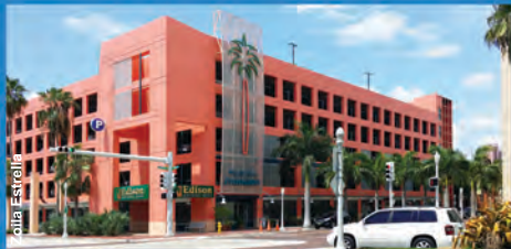
City of Palms Garage 2118 Bay Street - Bay & Monroe street entrances
