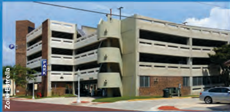
Main Street Garage 2286 Main Street - Main & Second street entrances
